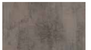
CONCRETE METALLIC OXIDE
